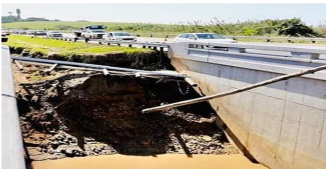
Figure 1: Mhlali bridge on N2 road (Source: The north coast courier)
