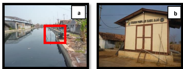
Figure 2: (a) Water pumps to dispose of inundated water from floods into the Bremsi River (b) Water pumps to dispose of inundated water flooding into the Meduri River (Rosida, October 13, 2018)
