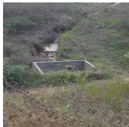
Plate 3: Lower Course of Antorun Reservoir Showing the Excess Water Outlet
